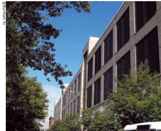
Morgan Mail Processing Center Outfitted with Opaque Film over the Glass to Prevent Bird Strikes
